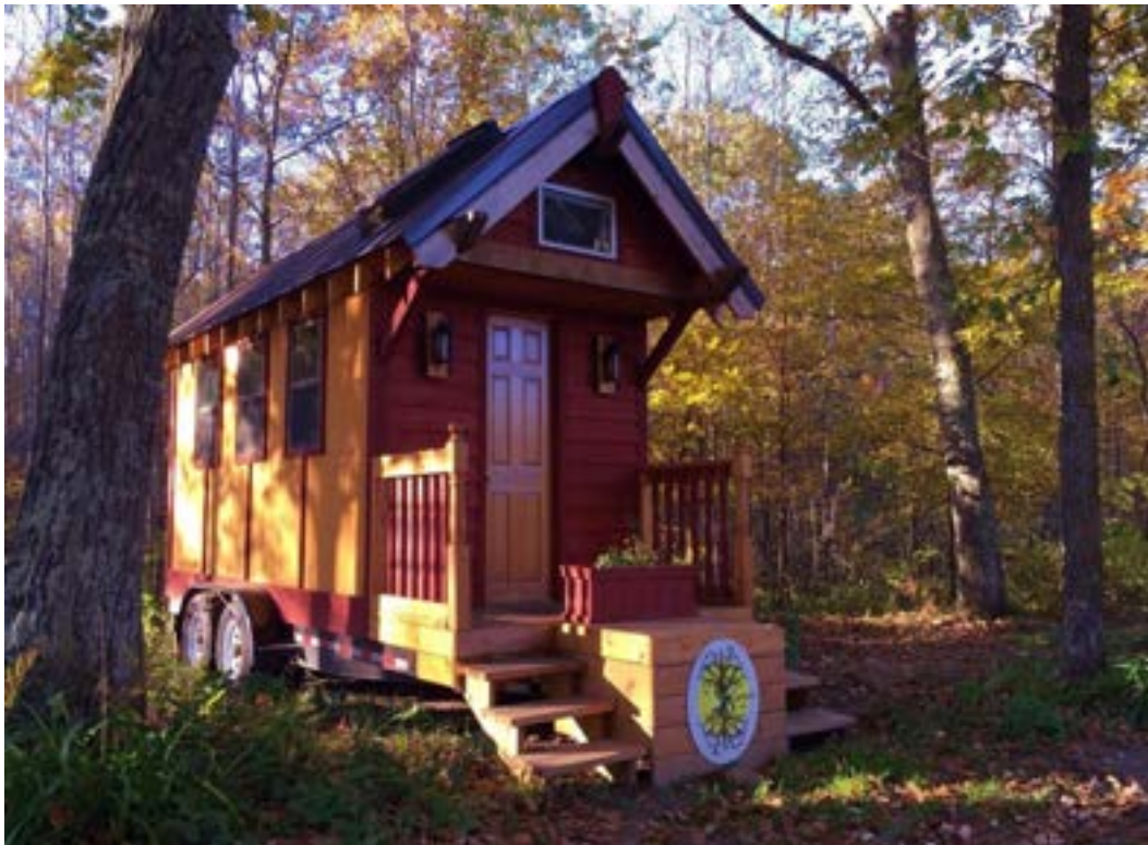
Figure 4 “Tiny home at the Sanctuary Minnesota. From The Sanctuary Minnesota , n.d., https://www.thesanctuaryminnesota.com/new-gallery .
