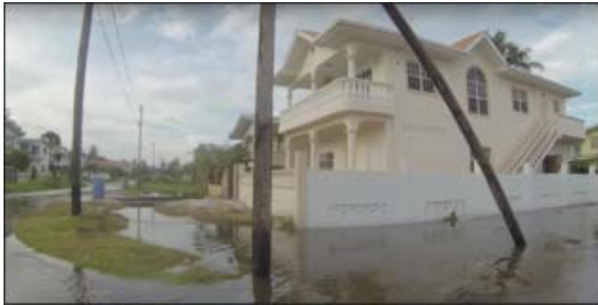
Figure 5 Screenshot of electrical poles in Georgetown becoming rotted by floodwater. From The Real Atlantis – Is Georgetown, Guyana a Sinking City? (7:18), by Real Guyana, 2013.
