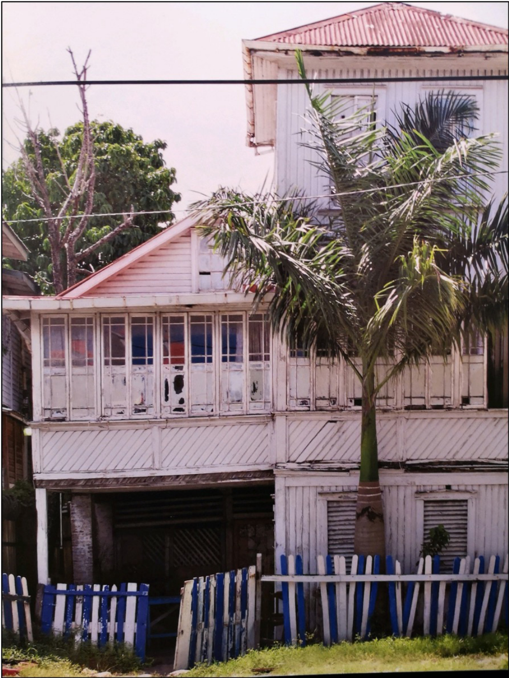
Figure 3 A house in Georgetown built in a colonial architectural style. From City of Wooden Houses (p. 49), by C. Davis, 2017, Merrell Publishers. Copyright 2017 by Merrell Publishers.
