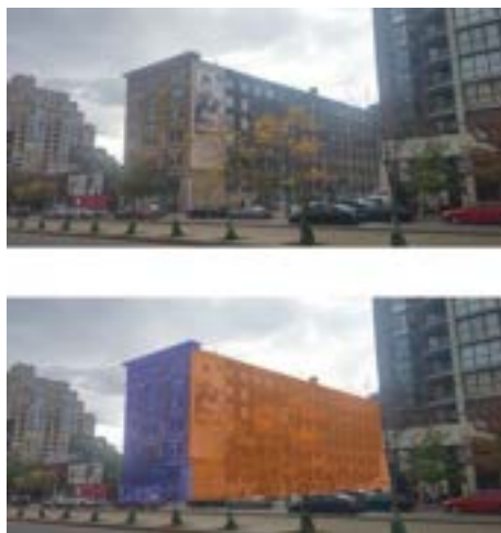
Figure 7. The front façades (blue) have been restored to a much higher degree than the rest of the structures (orange), producing a consistent historic street wall along Spadina that presents a superficial image of a pristine and immaculately restored neighborhood.
